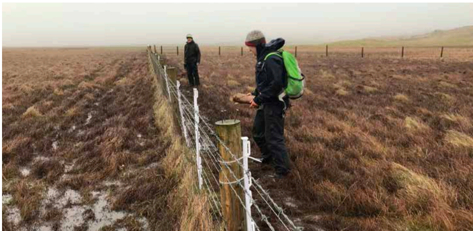
Predator fence installation
