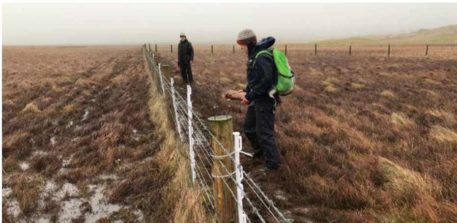
Predator fence installation
